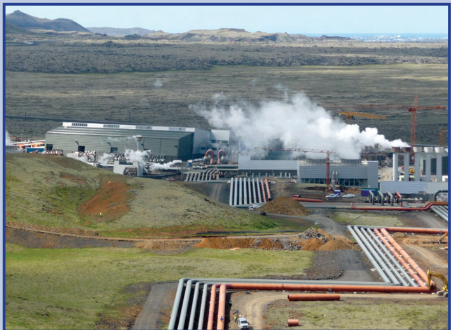
Geo-thermal Power Plant at Hellisheidi, Iceland
